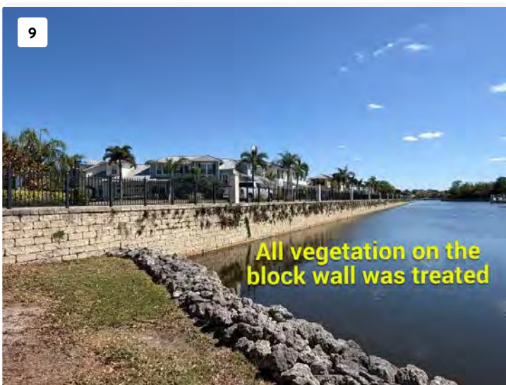
Block wall along Cafrey Place
